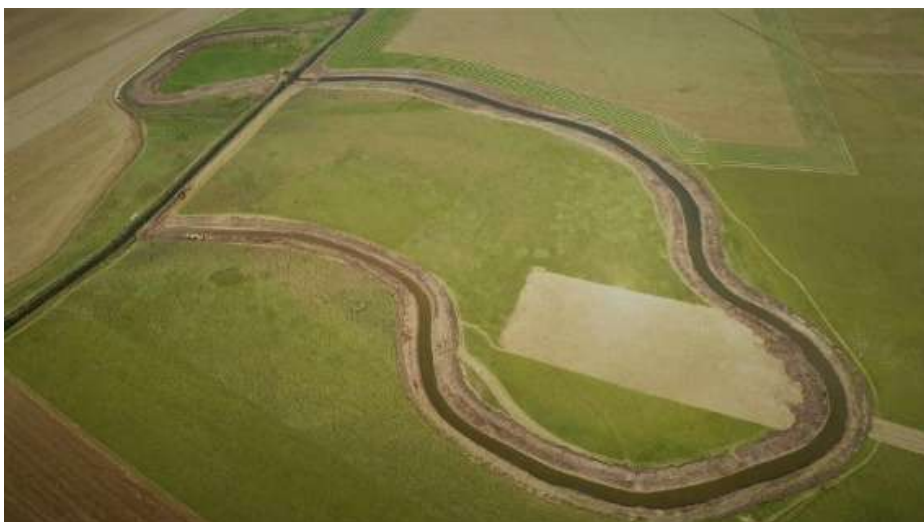
Fig. 1 Aerial view of the restored double meander and artificial straight channel of Stržen
