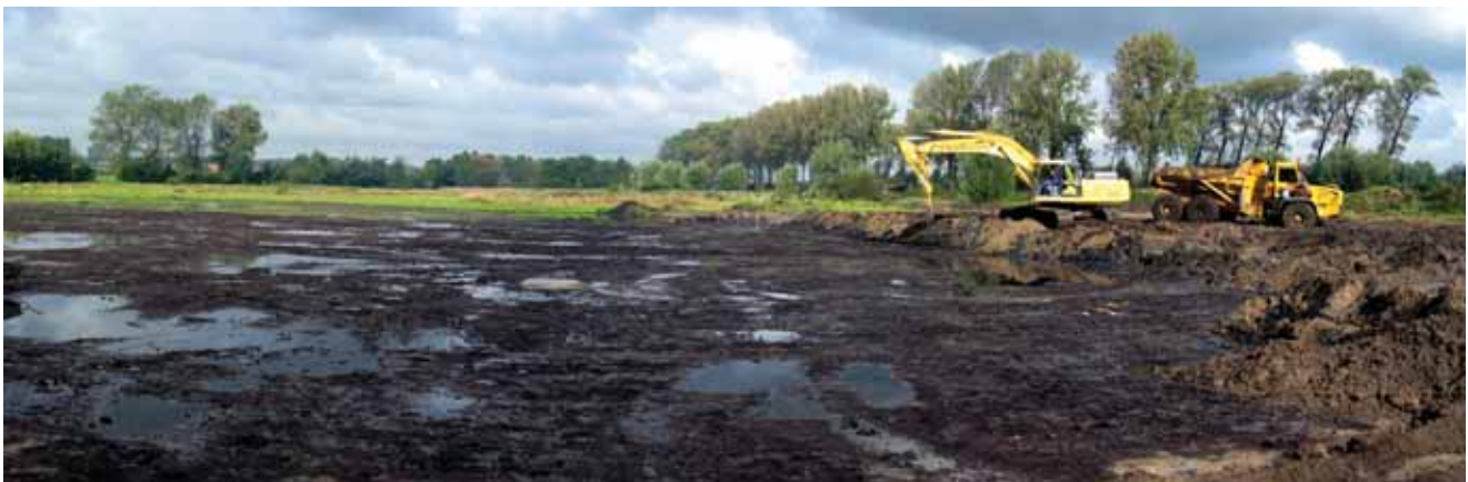
Removal of the sludge down to the original peat soil.
