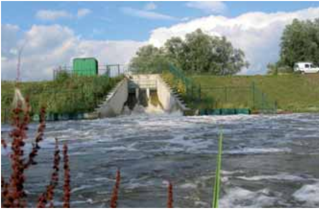
Detail of the inlet sluices in the dike during flood when water is entering the FCA-CRT Lippensbroek.
